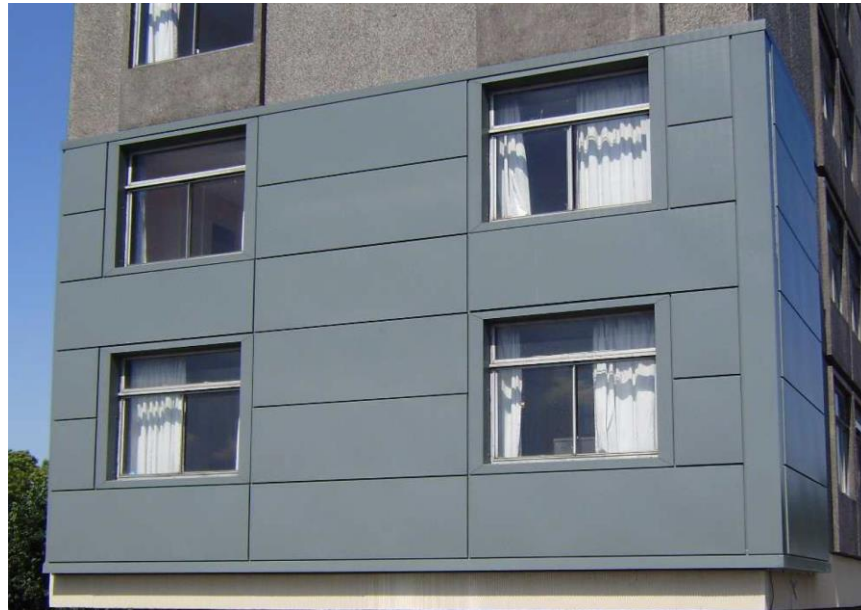
Figure 5. Building facade renovated with UTC panels [14].
