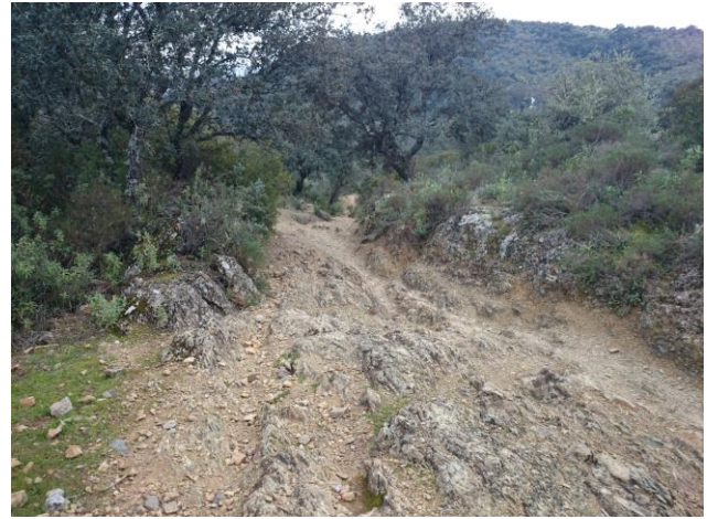
Fig. 5: Structure of the rock-cut road between Córdoba and Loma de los Escalones (Antonio Monterroso for © Project Ager Mellariensis).
