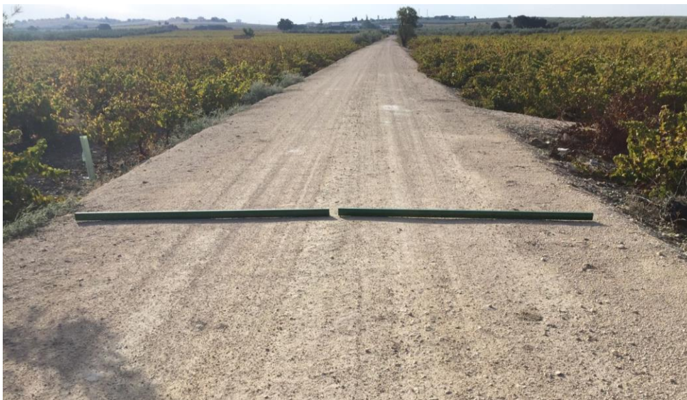
Figure 5.5: Straight edge of 2 m in each wheel path.
