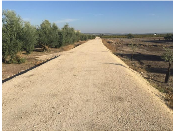
Figure 5.2: Section III of experimental unpaved rural road.
