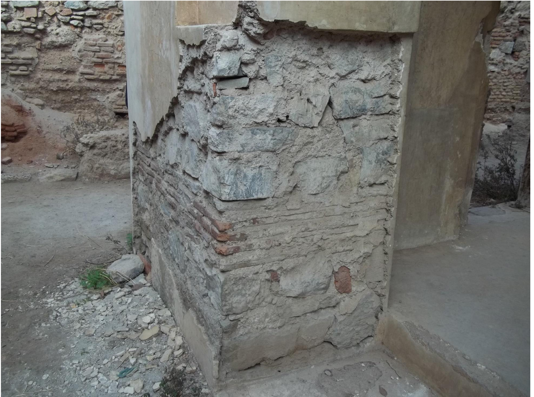
Detail of the stone and brick work
