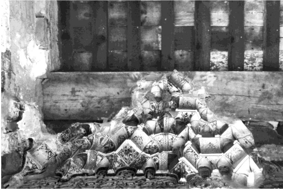
Fig. 7: Granada, Alhambra, Comares courtyard, south-west alcove, remains of a muqarnas vault. The medina is decorated with interlaced strapwork. (photo M. Massaiu).
