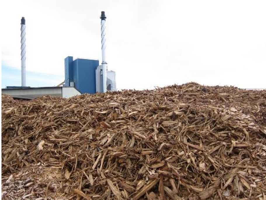
Figure I-4. Biomass conversion plant.
