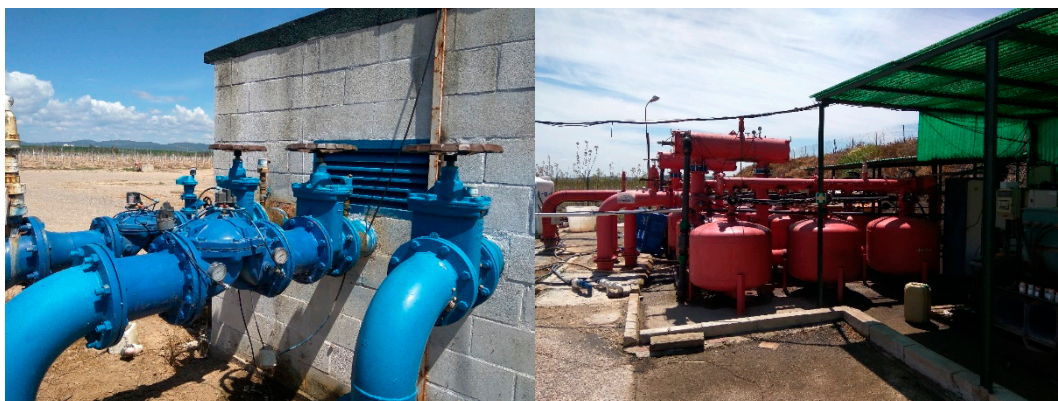
Figure 2. Hydrant and filter plant where the HPP will be installed.
