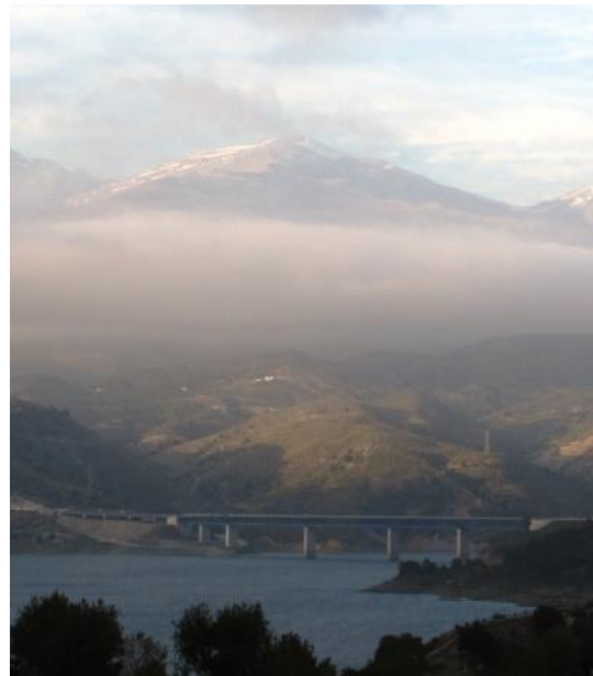
(b) Reservoirs presence for water optimisation engineering solutions
