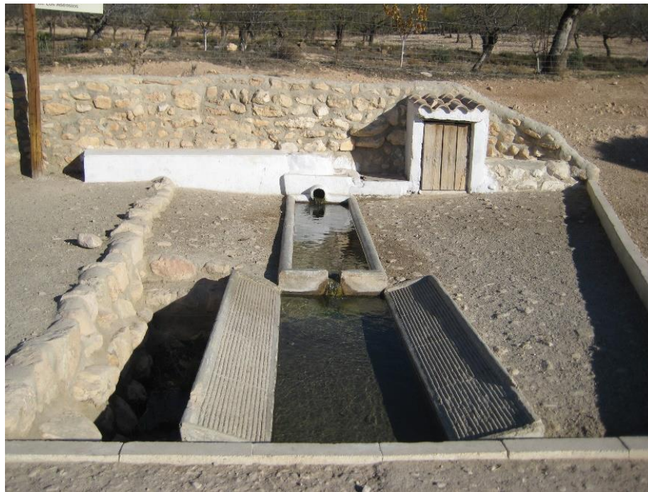
45 Fig.1 Drinking trough and washing space at the end of the qanat's pithead in Fuente 46 Grande (Los Vélez, Almería) 47 48 49
