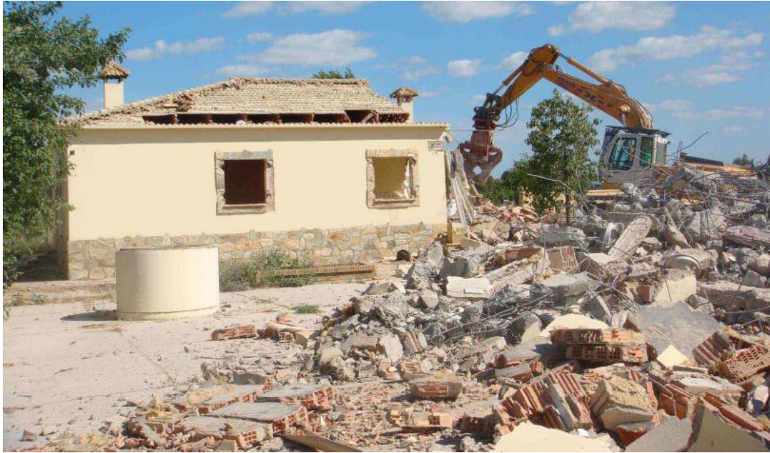
Fig. 2. Selective Demolition of single family homes
