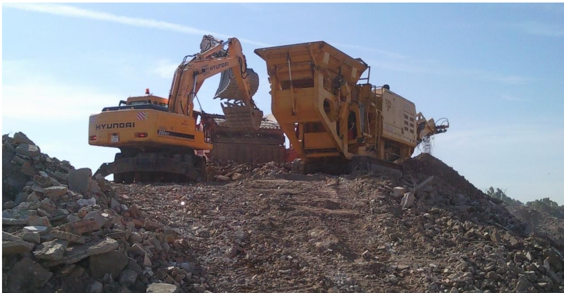
Fig. 3. Mobile Plant: Aggregate Screen and Jaw crusher.
