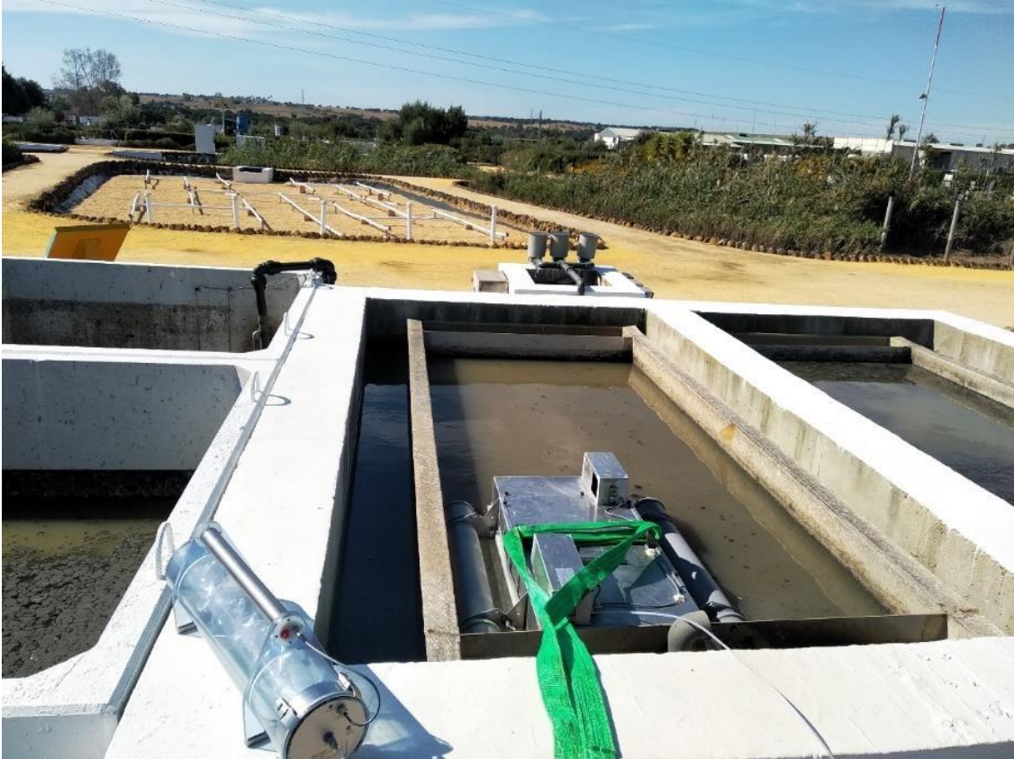
Figura 40. Tanque Imhoff.
