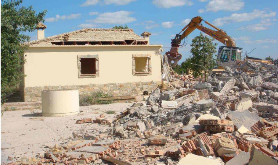
Fig. 5-2. Selective Demolition of single family homes
