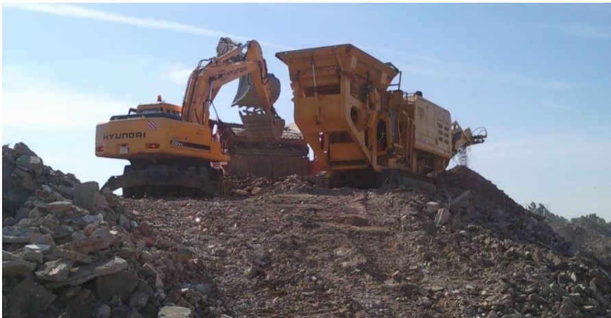
Fig. 5-3. Mobile Plant: Aggregate Screen and Jaw crusher.
