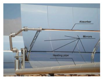
**Figure 3.** Detail of a cylindrical-parabolic solar collector of a Solar Thermal Power Station (photo by T.J. Teleszewski).
