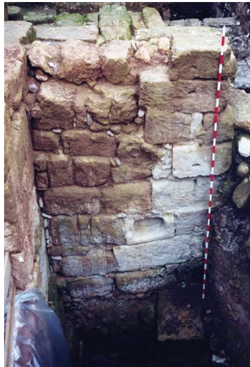
Figure 6. Structures of the early Emiral period (8th century) in the Patio de Mujeres del Alcázar de los Reyes Cristianos (Women’s Courtyard of the Christian Monarchs’ Fortress), consisting of the regularisation of the former urban wall line made with reused materials (image: GMU-UCO Agreement).
