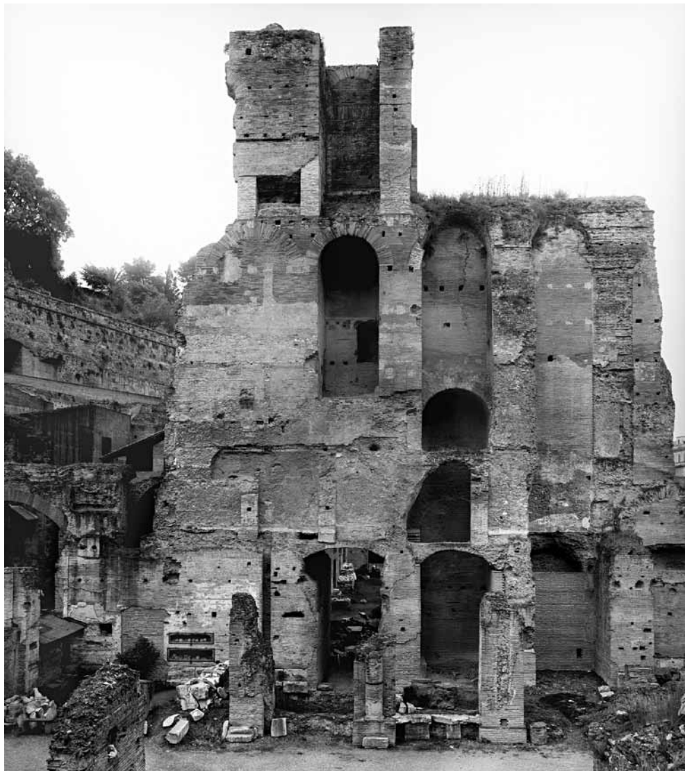
FIG. 6: North façade of western hall (DAI Neg. Nr. 42.897)
