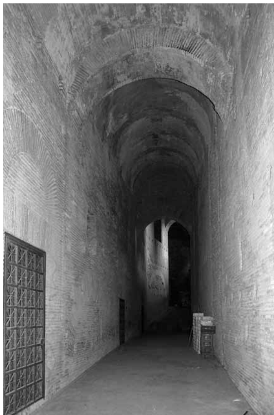
FIG. 12: Ramp, ground floor looking west (author).
