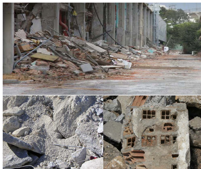
Fig. 1. Demolition of the Ciatesa factory (Málaga).
