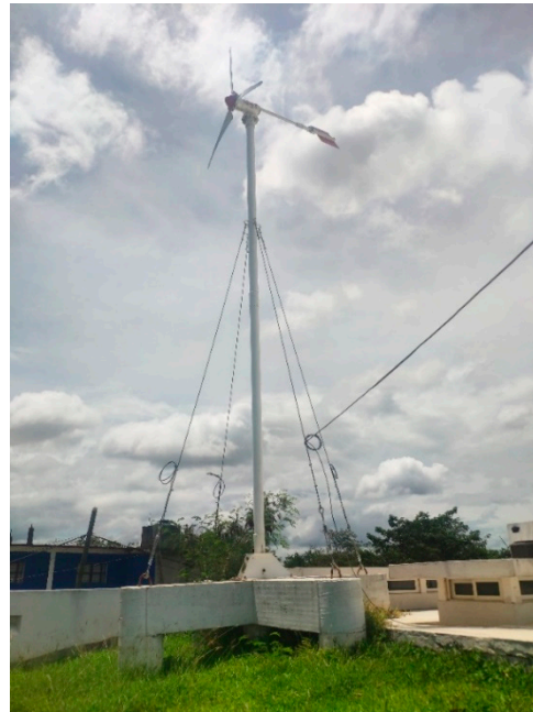
Figure 1. RTO-1kW Wind Turbine, installed in the Ejidal Bioclimatic Community Center of La Venta, Oaxaca, Mexico.
